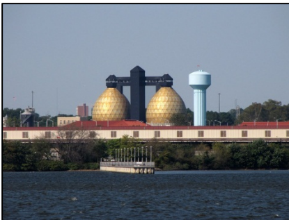
Back River Wastewater Treatment Plant
