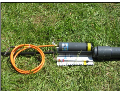
Extensometer Instrumentation for WSSC Bi-County Water Tunnel
