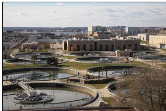
DC WATER Blue Plains Enhanced Nitrogen Removal Plant
