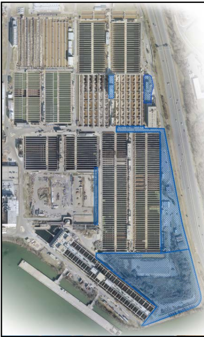
DC WATER Blue Plains Enhanced Nitrogen Removal Plant
