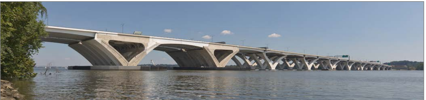
Woodrow Wilson Bridge
