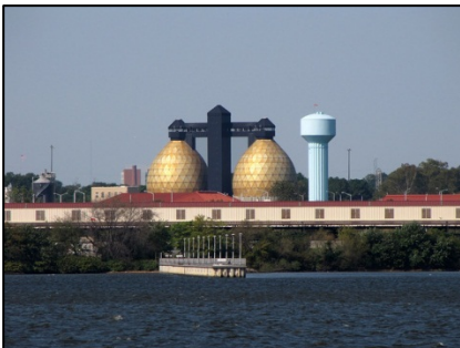
Back River Wastewater Treatment Plant
