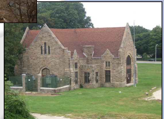
Ashburton Pump House
