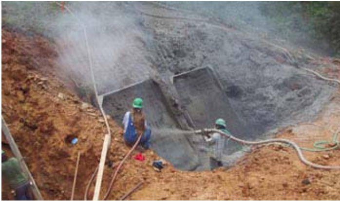
Workers are spraying shotcrete for one of the pads.
