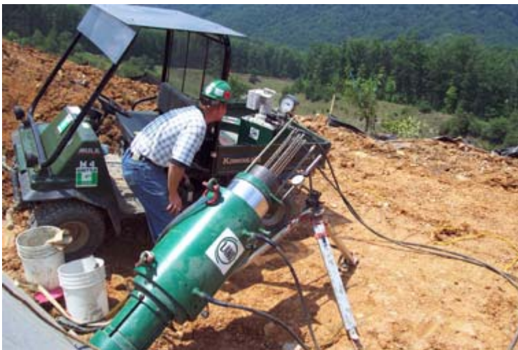
Proof loading an installed ground anchor.
